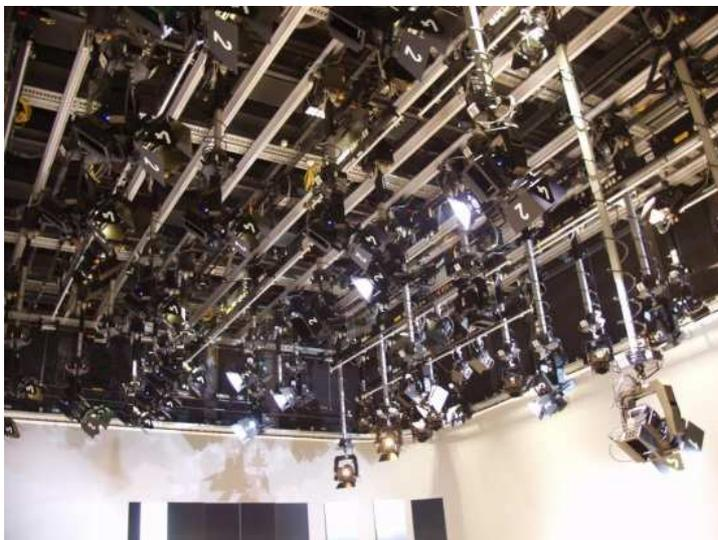
Ceiling construction system with rails, hoists und luminaires
