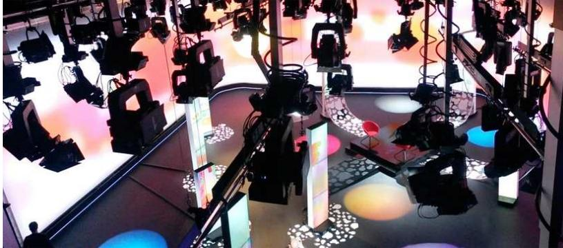
View from the gallery: telescopes with LED luminaires, barrel hoists with effect light and LED background lighting
