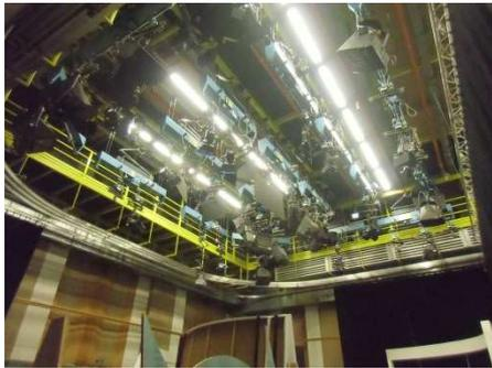
Old studio lighting technology with barrel hoists and pantographs
