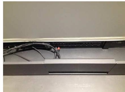
Floor canal with sockets and instruments for wiring to the playing area
